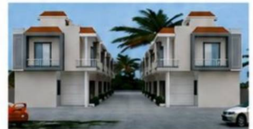
Internal RCC Road
